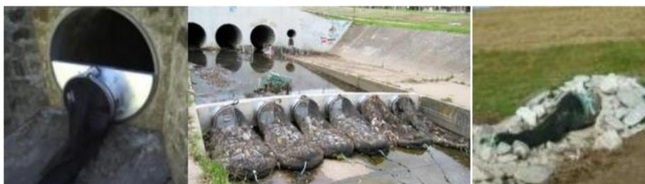
Filets sur exutoires (<http://stormwatersystems.com/stormx-netting-trash-trap/>)
